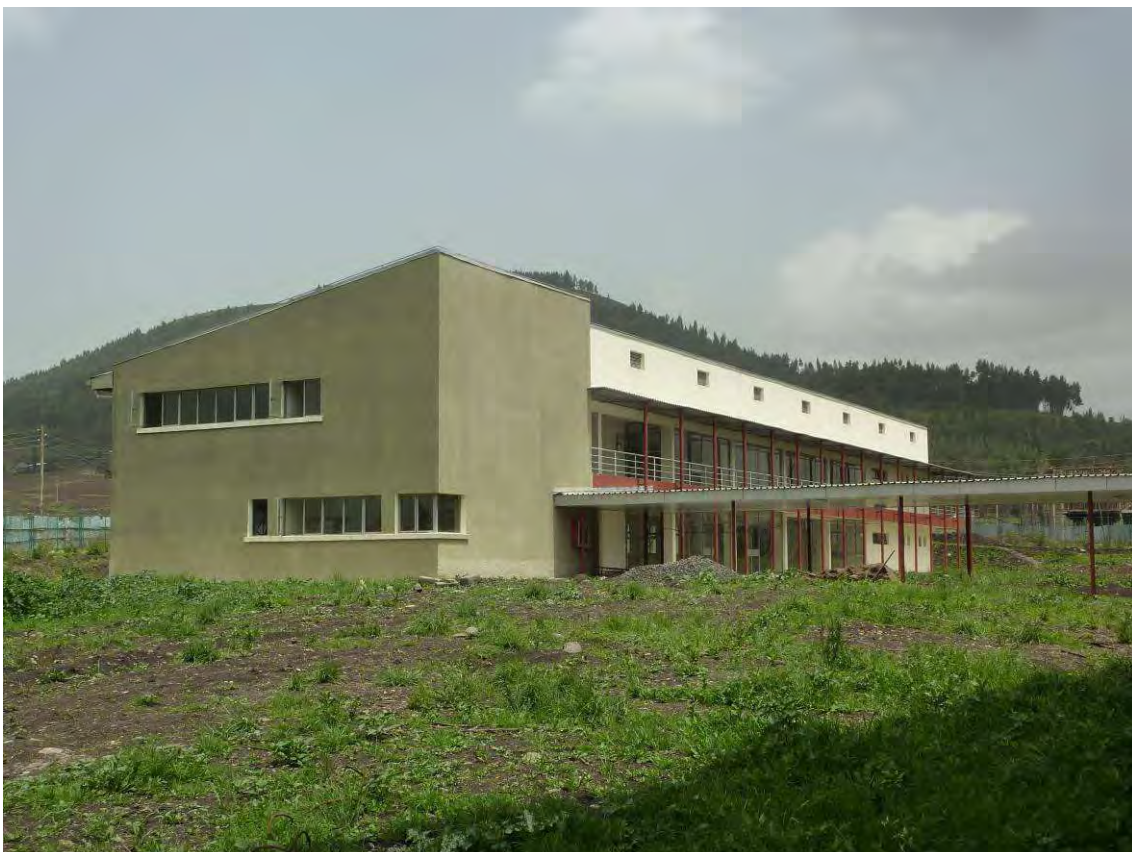
Service Centre (A),finished for 90%.
