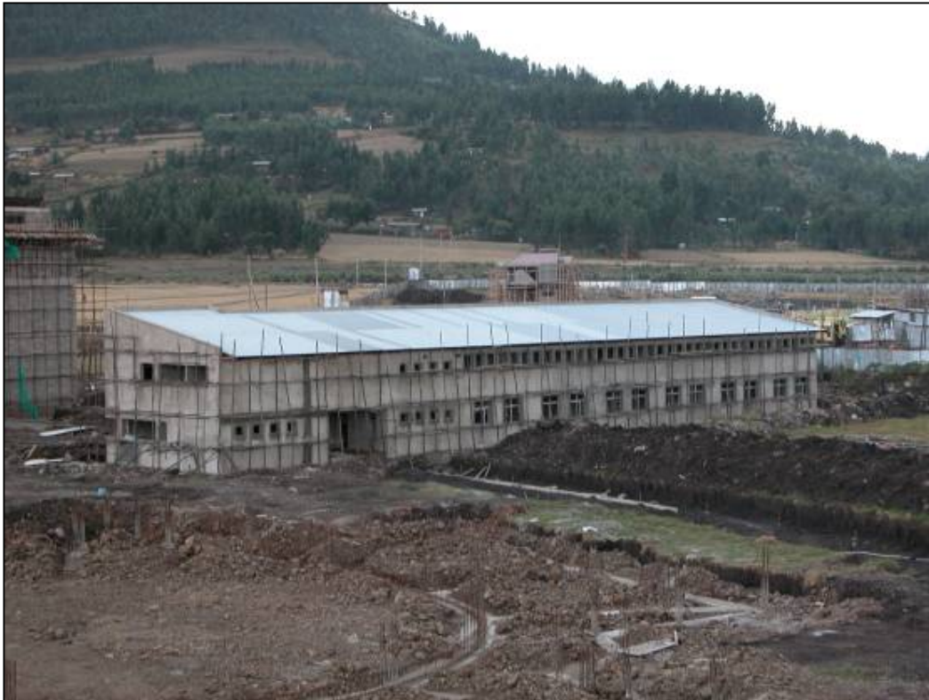
Administration Building (C)
