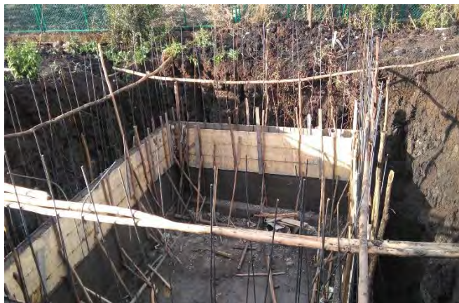
a) initial stage of the new sewerage tank
