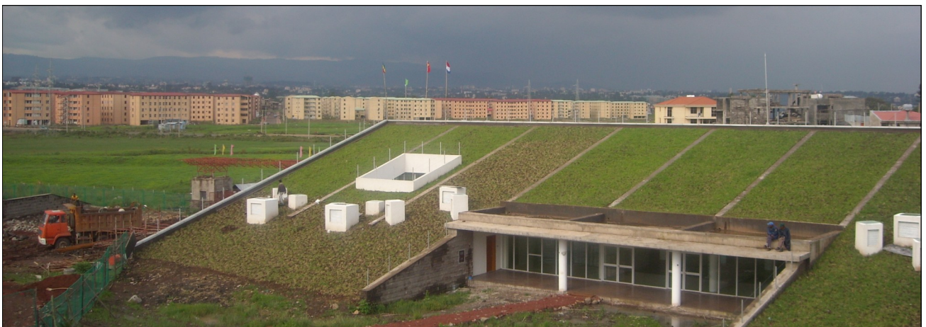
New grass on the roof of the De Pagter Library
